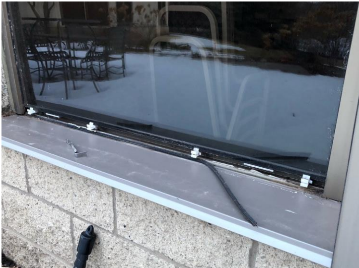
Figure 3 - the frame of the windows did not incorporate a sill pan to direct water to the exterior. The flashing shown stops at the front of the window where it met the gasketing and no end dams were incorporated. Also evident is the previous attempt to seal from the outside where the flashing meets the gasketing. (Photo courtesy Inspec)
