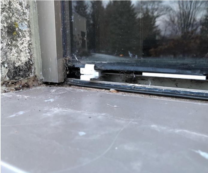
Figure 2. Plastic clips secure the aluminum to the glazing gaskets, allowing movement and water entry. (Courtesy Inspec)
