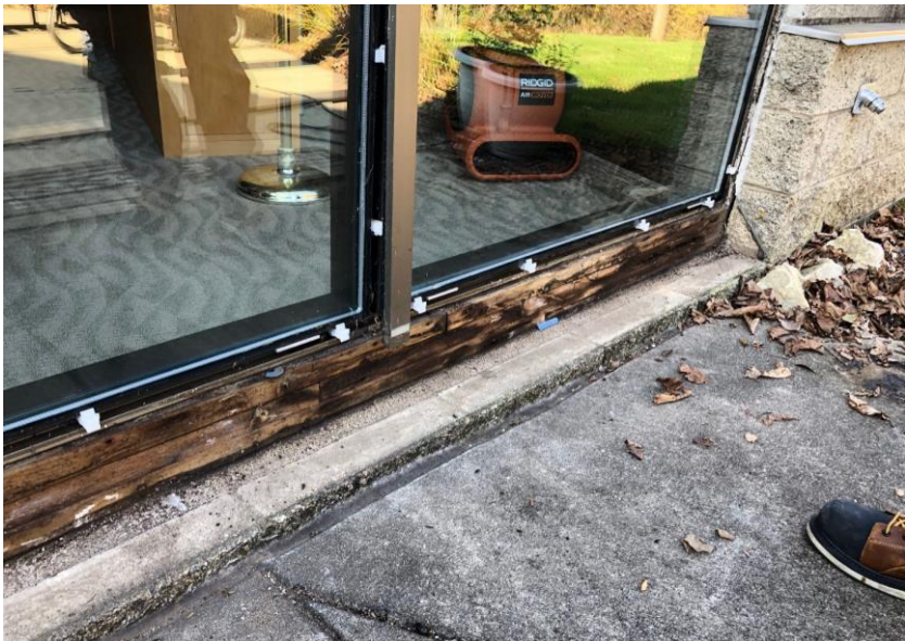
Figure 5 – Storefront system lacking proper sill pan and end dams allowed water to escape into the wall below the sill, causing damage to stacked wood framing. (Courtesy Inspec)
