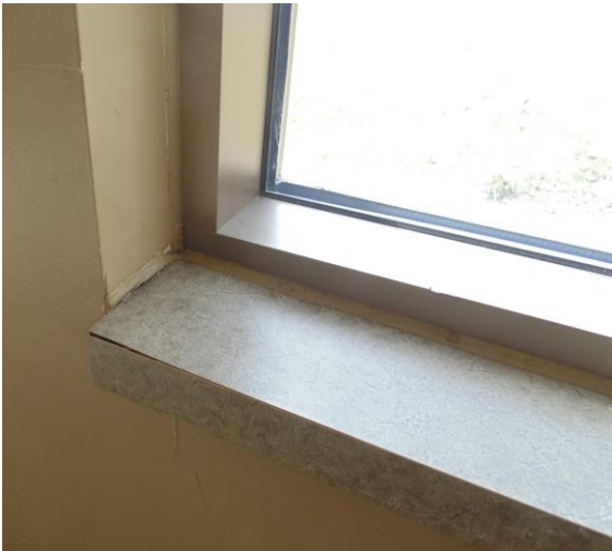
Figure 1. Visible moisture damage of the plastic laminate sills . (Courtesy Inspec)
