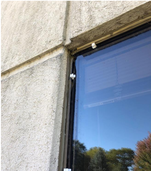
Figure 3 - the frame of the windows did not incorporate a sill pan to direct water to the exterior. The flashing shown stops at the front of the window where it met the gasketing and no end dams were incorporated. Also evident is the previous attempt to seal from the outside where the flashing meets the gasketing. (Photo courtesy Inspec)
